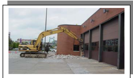
Concrete replacement project at Central Fire Station in September 2007 (above)
