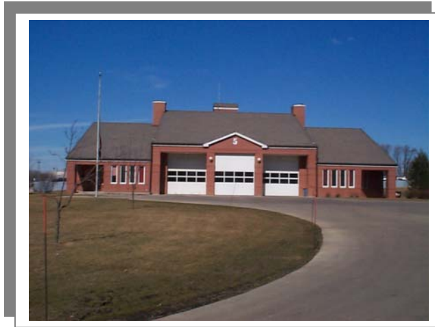
Station 5 730 Hill Avenue (630) 851-2825 Battalion 1 Headquarters
