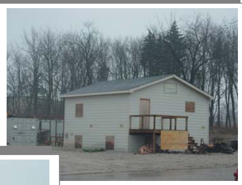
Pictured above: Structural Collapse House
